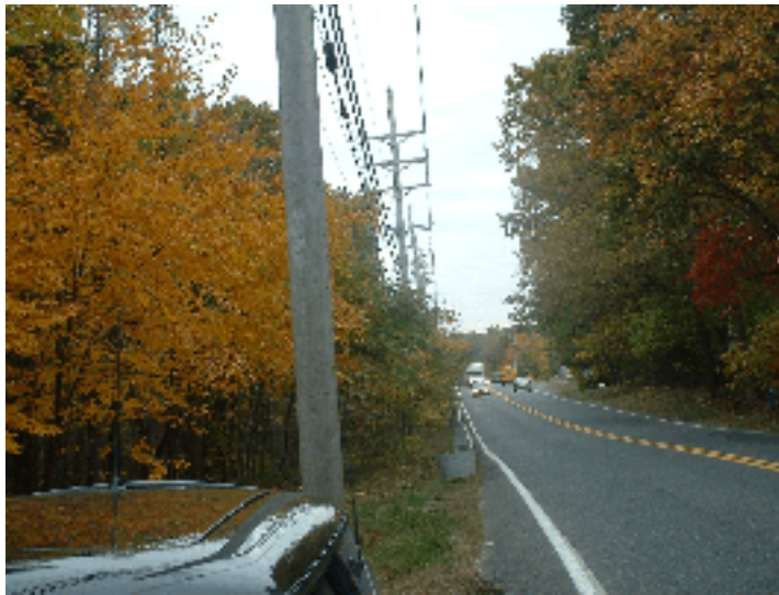
Looking southwest on Route 537 from the intersection of Route 537 and Paint Island Spring Road
